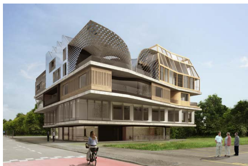
NEST testing facility at Empa
